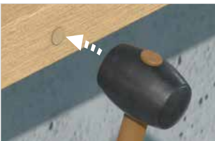
Hammer in plug with rubber mallet
